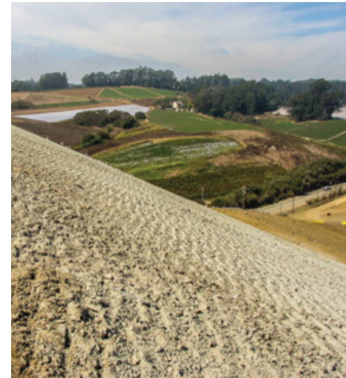
Posi-Shell Intermediate Cover on thin soil leveling layer
