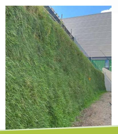
The combination of these components results in a vegetated wall system that integrates seamlessly into natural landscapes. By supporting rapid plant establishment and sustained growth, Rootlok contributes to increased biodiversity and complements the local environment. Its environmentally friendly materials and design make it a preferred choice for projects aiming to enhance green infrastructure and promote ecological balance.
