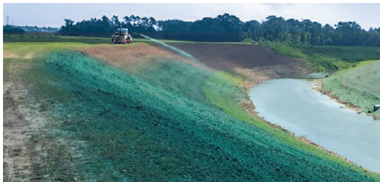
Before: The site was sprayed with EarthGuard® Fiber Matrix™ just before the hurricane as part of a regular erosion control maintenance plan. 8/24/17
